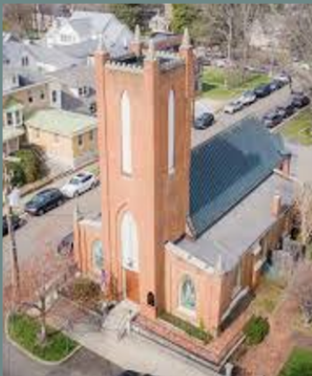
Aerial view of current building. Differences in brick on the sides of the tower illustrate where the original roof was and the sides show where the roof was lowered.
