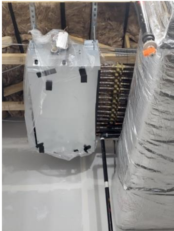
Unit inside that distributes refrigerant to each room in the building
